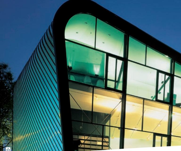
Aluminium has become an increasingly popular choice for façade cladding in recent years. Alongside its low weight and outstanding mechanical characteristics, its most convincing aspect may well be the creative possibilities that it offers architects and building contractors. Aluminium is light, easily shaped and can be colour coated and processed in various ways. Reynolux® fulfils all these requirements in grand style.
